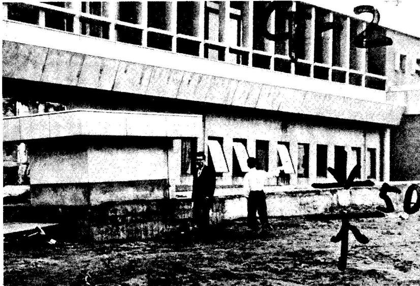
FIG. 5. GROUND SETTLEMENT DUE TO LIQUEFACTION (AFTER H. KAWASUMI, 1968).
