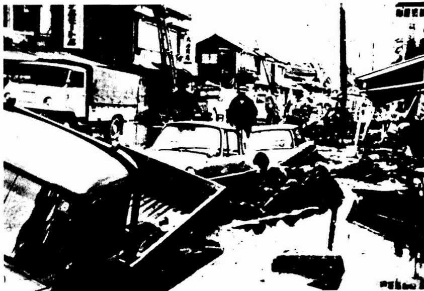
FIG. 14. NEWER NIIGATA AFTER EARTHQUAKE - GREAT DAMAGE DUE TO LIQUEFACTION OF RECENT DEPOSITS (AFTER H. KAWASUMI, 1968).
