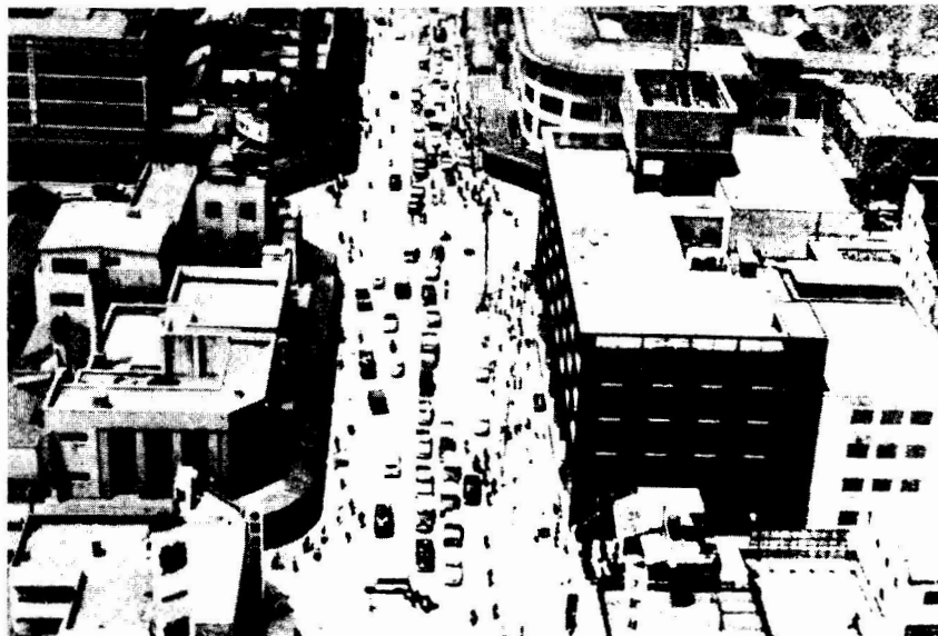
FIG. 13. OLD NIIGATA AFTER THE EARTHQUAKE - LITTLE DAMAGE ON OLDER DEPOSITS (AFTER H. KAWASUMI, 1968).
